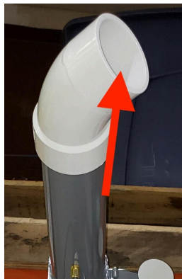
Figure 15) Protecting Fan Outlet From Animals
